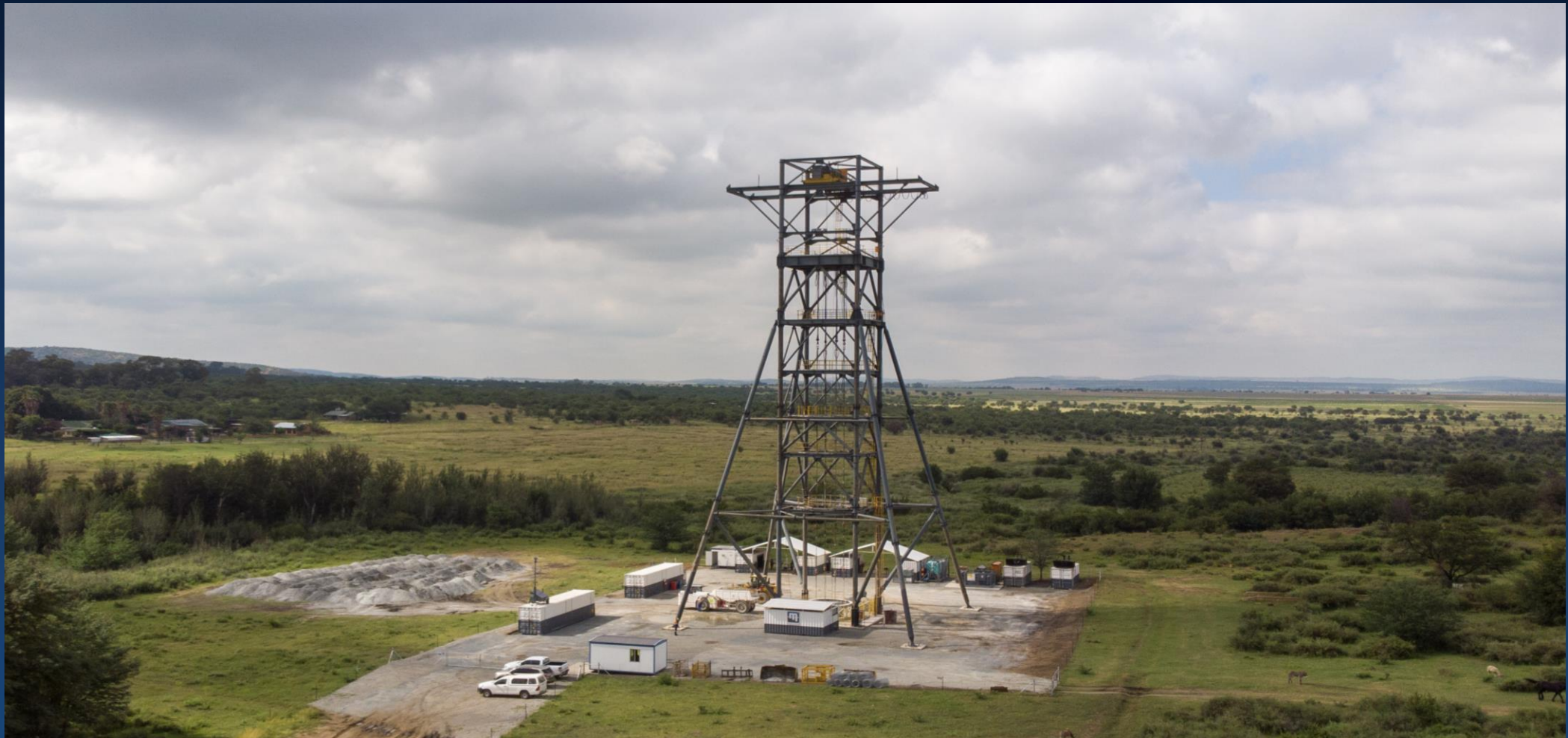
Image: SBS machine sunk through surface collar.
