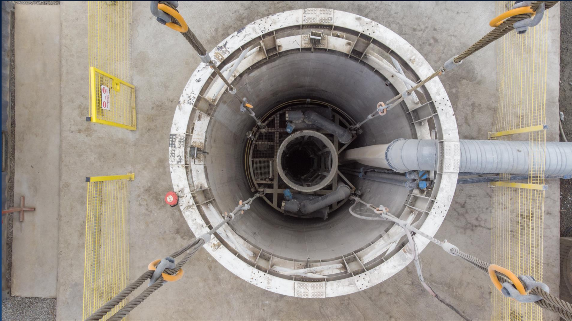
Image: SBS, 50m deep experimental shaft sink.
